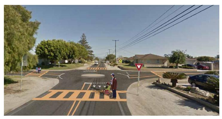
**CONCEPTUAL DESIGN ONLY:** Installing a mini roundabout slows vehicles down in this minor intersection. The center "island" can now be used for public art or other community identifier.
